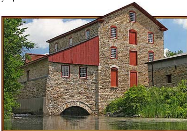
The Old Stone Mill in Delta Ontario, built in 1810, showcases milling technology and 1800s industrial heritage.
